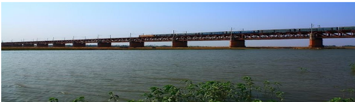
Abdul Bari Rail-Cum-Road Bridge (Koilwar Bridge) on Sone River connecting Patna District to Bhojpur District (Ara)
